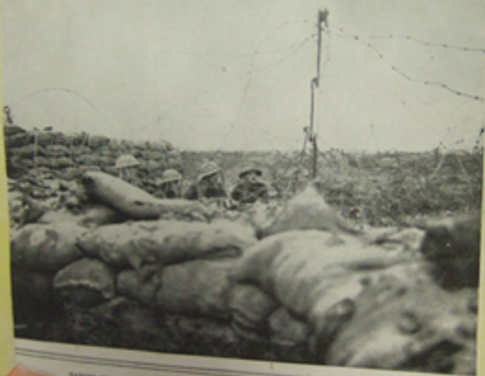
BARBED WIRE DEFENCES ARE NOW CONSTRUCTED; ENTANGLEMENTS WITH IRON POSTS BEFORE A BRITISH FRONT LINE TRENCH.
