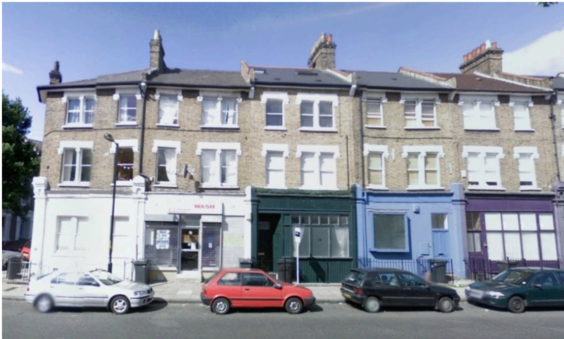
Figure 74. Type F (min. cost £500), Houses with shops, Denmark Road
