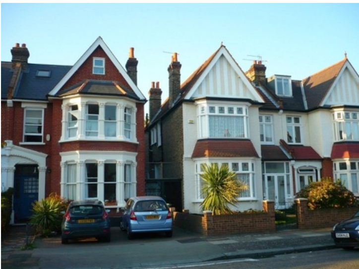
Figure 169. Houses in Arran Road built by James Watt. On the left the 'older' style, on the right the 'newer' style but otherwise the same configuration and layout.
