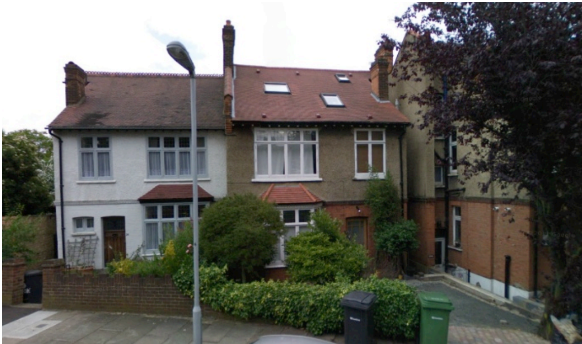
Figure 215. Dunoon Road, built by Charles Walker, 1906, blockplans only by Stone
