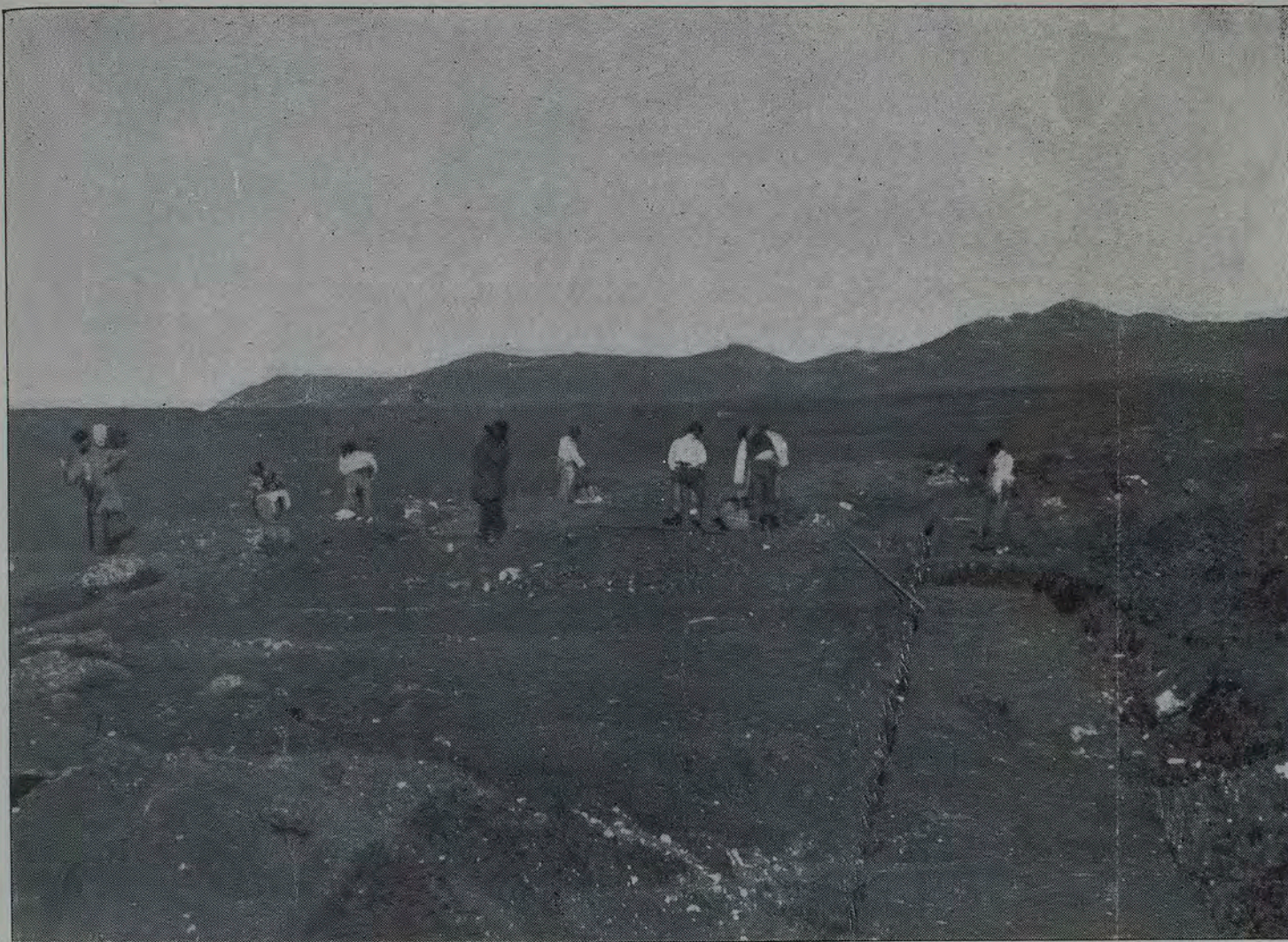
NO. 1.—WALL K, LOOKING EAST.
