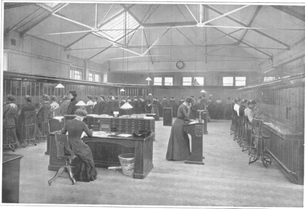
IN THE POST OFFICE CENTRAL TELEPHONE EXCHANGE (ST. PAUL'S CHURCHYARD): RECEIVING CALLS.
