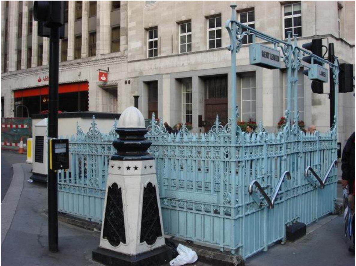
Figure 4.1 Eastcheap Underground Public Conveniences, City of London
