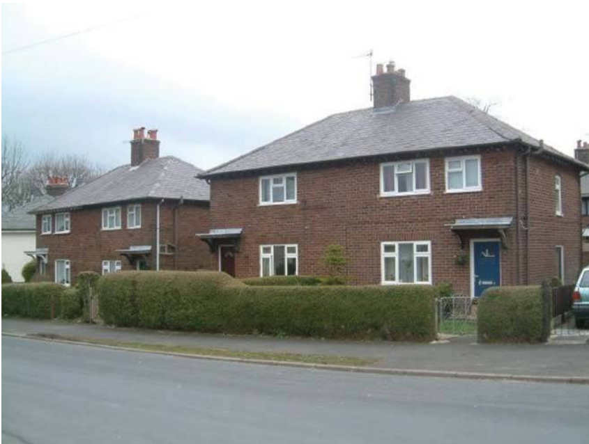
FIGURE 2 Sherwood Road (Heath Grove Site), built 1926. After the erection of the Cliff Road houses, which were uniquely designed but criticised on an aesthetic and cost basis, the Buxton council resolved to use the now widely familiar designs as provided by the ministry of health for the rest of the town's schemes.
