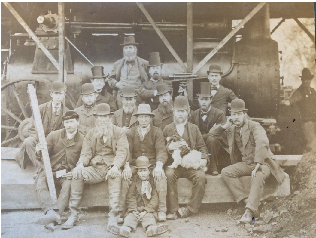
Figure 10 Beside the Steam Engine at Chiswick's Sewerage Pumping Station. 43
