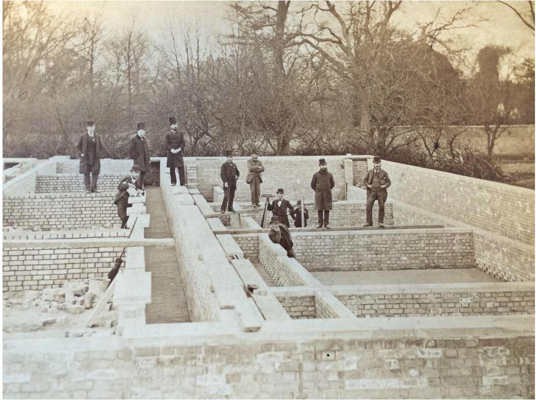
Figure 9 A visit to Chiswick Sewerage Works' Filter Tanks at Corney Reach. 42
