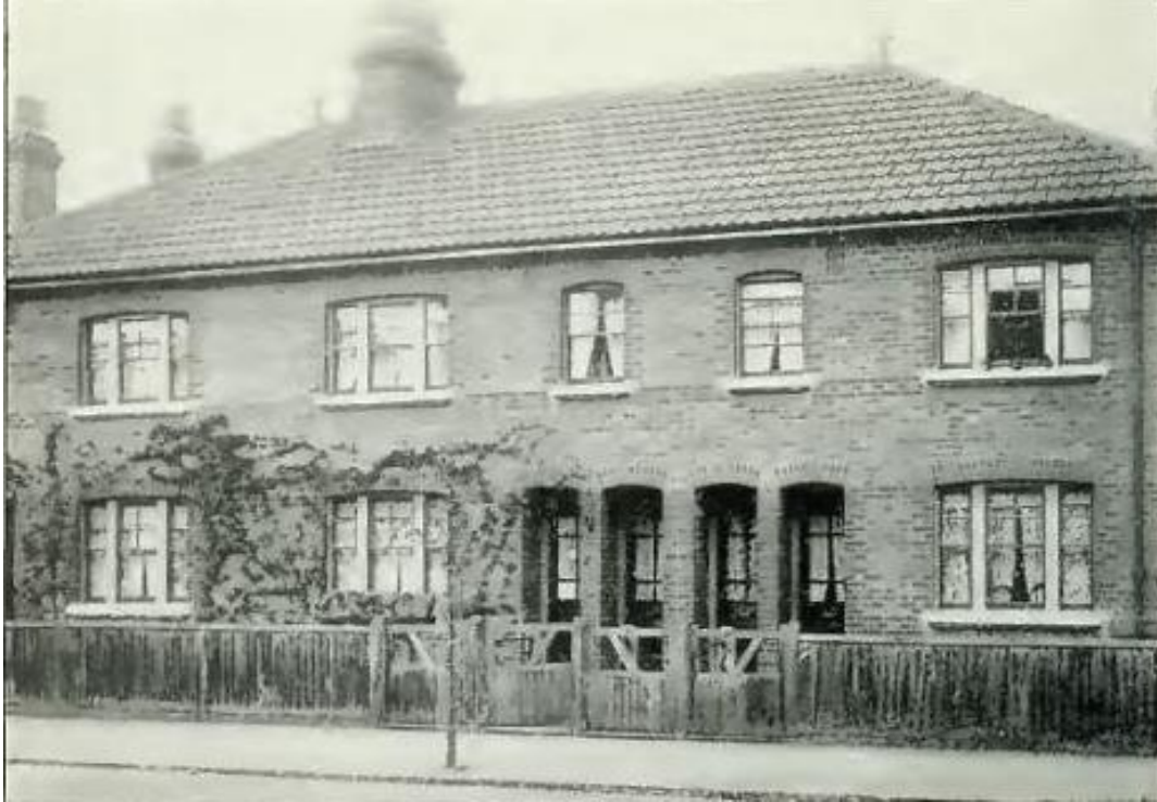
Illustration 2.8: Municipal tenements, or 'cottage flats' in Richmond at Manor Grove. 104
