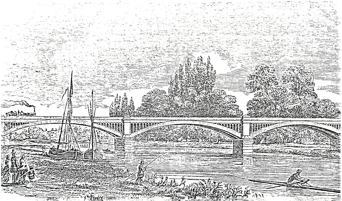
Illustration 1.6: The Richmond, Windsor and Staines railway, the bridge at Richmond. 76
