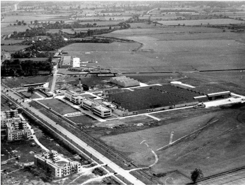
Fig 8 Aerial view of development (BAe Archive)
