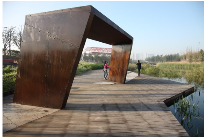
Figures 96. Rivetted recycled steel in walkways or bent to frame a view (Turenscape, http://landezine.com/index.php/2011/02/shanghai-houtan-park-by-turenscape/ [Accessed 30 June 2020])
