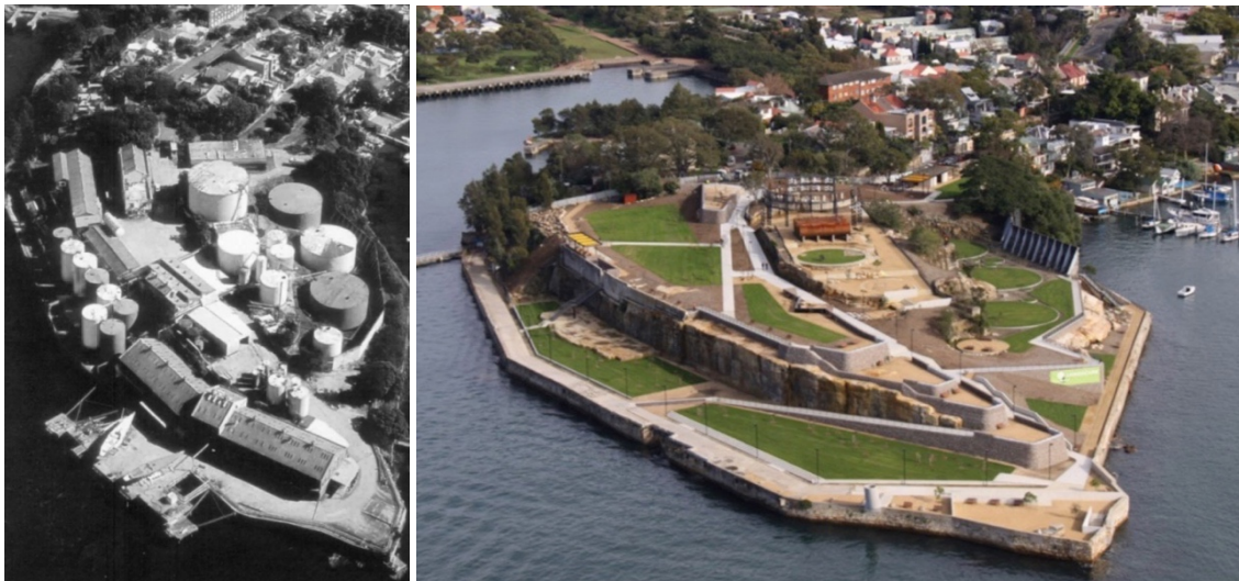
Figures 12-13. The original site in 2002, and as it is now (Sydney Harbour Foreshore Authority, http://www.shfa.nsw.gov.au/content/library/documents/DF93B680-DA31-C0D8-88ADBF85C8806537.pdf and https://mcgregorcoxall.com/project-detail/125 [Accessed 20 March 2020])
