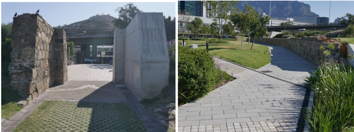
Figures 25-26. Contrasting original and new entrance walls, gate tracks embedded between them (Author, February 2020)
