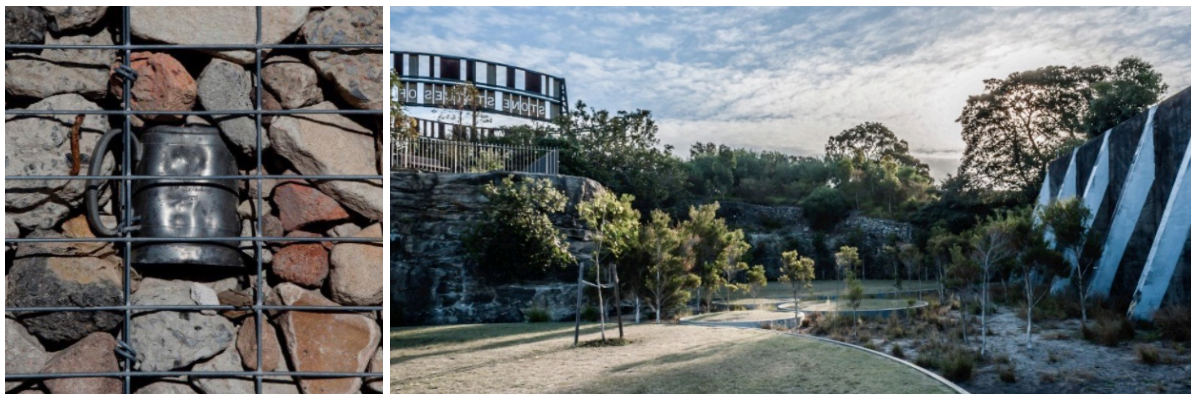
Figures 18. Old tankard from the former villa embedded in rubble filled gabion Figure 19. Two opposing walls, one original, one coloured by recycled coal waste surround grass tank circles ( https://mcgregorcoxall.com/project-detail/125 )
