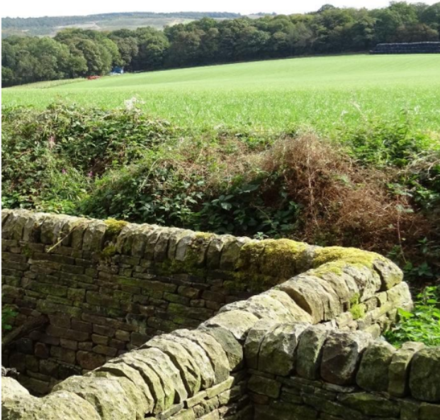
Figure 9. Hanging Trees , evidence of algae and moss on the stone wall (September 2019).
