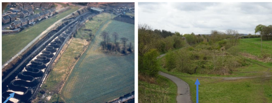
Lambton earthwork fabricated in coal spoil.
