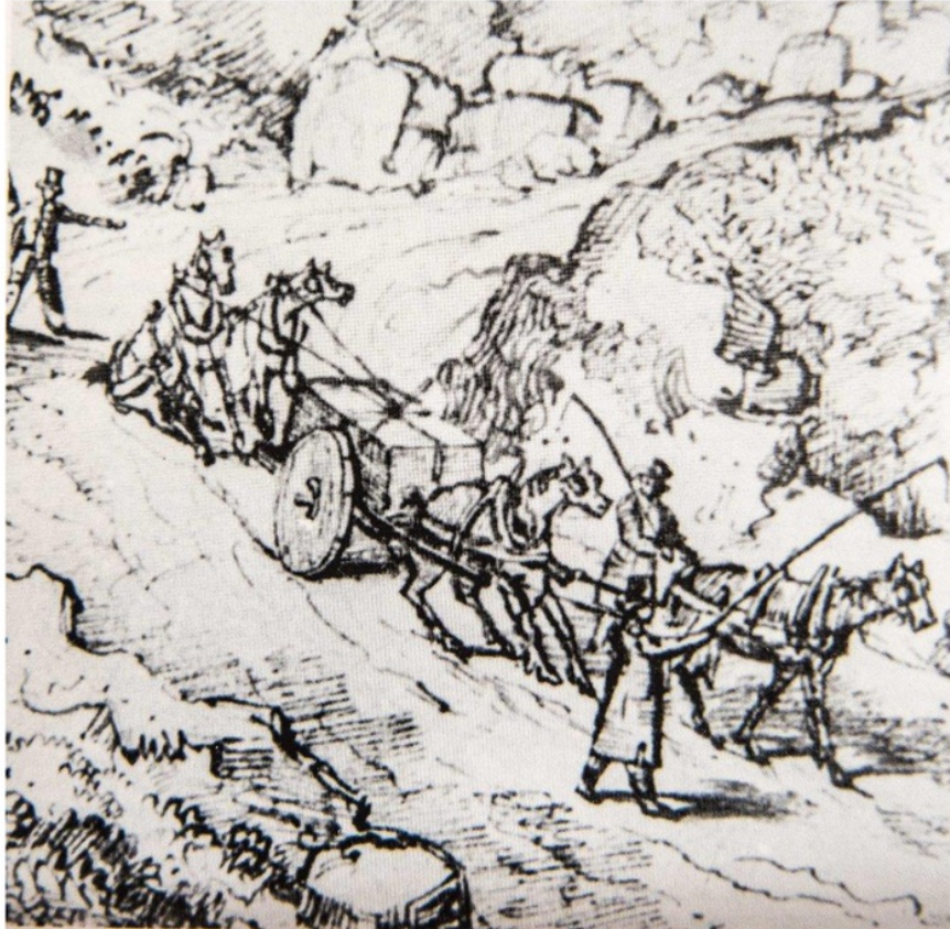
Figure 36. Transporting Portland stone by road in 1805 using a two-wheeled 'jack'. Horses at the rear acted as the braking system. This method was superseded by the steam driven traction engine later in the century.
