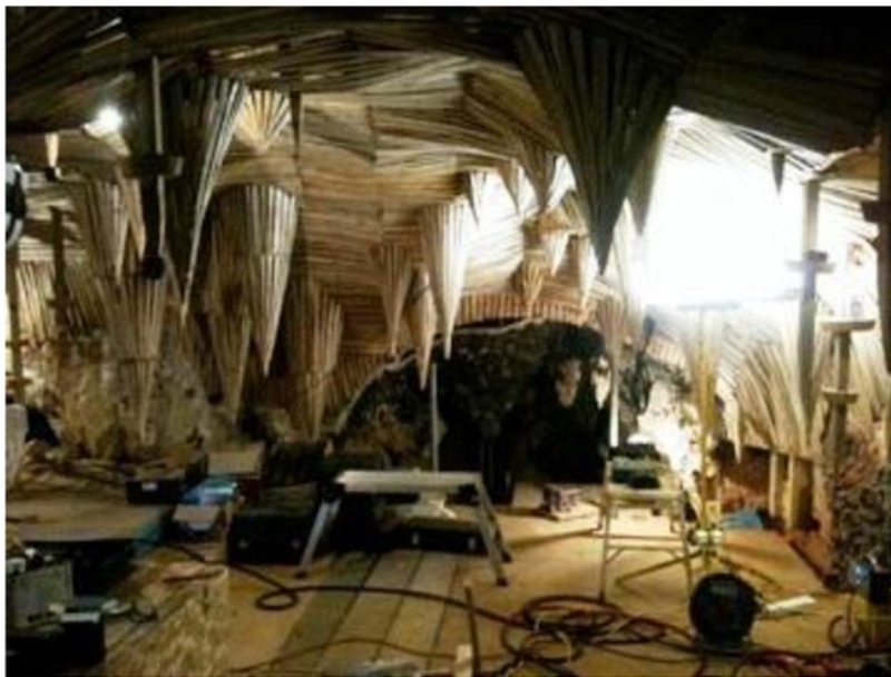
Figure 73. Wooden formers used in the reconstruction of stalactites at Painshill.
