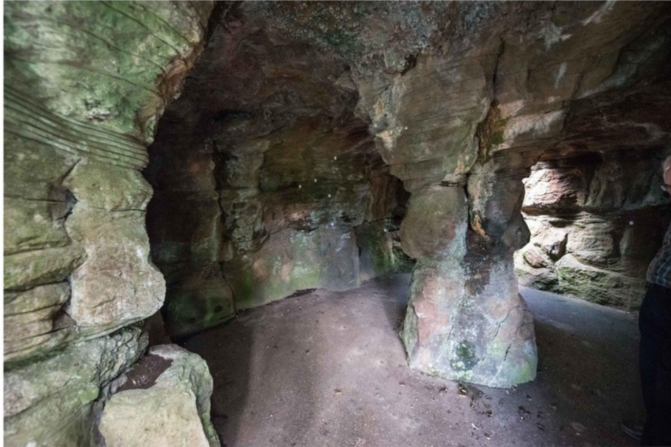
Figure 9. Undecorated grotto at Wotton House, made from pulhamite.
