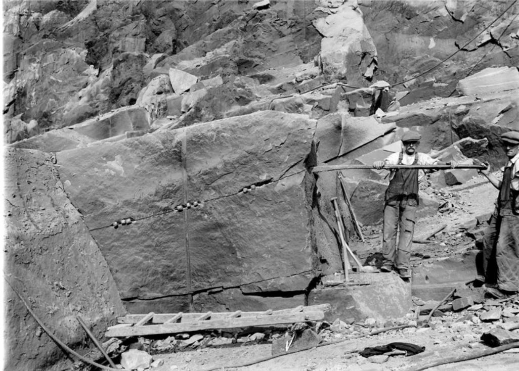
Figure 18. Splitting rock using wedges and lever.
