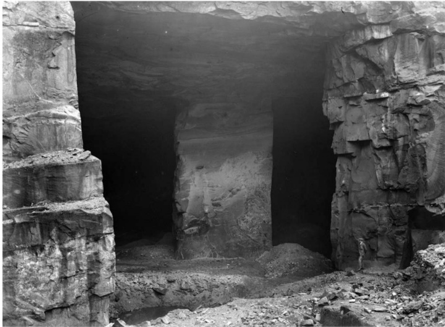
Figure 23. Pillar and stall method at Huntershill Quarry, Glasgow.
