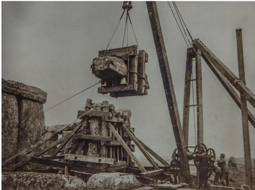
Figure 88. Stonehenge – 10-ton lintel being lifted by hand crane in 1920.
