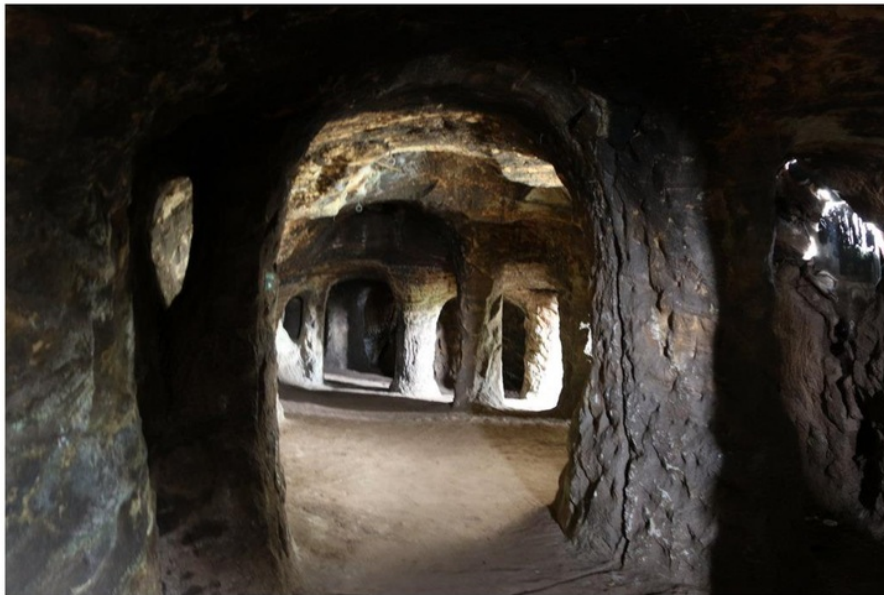
Figure 54. Hawkstone Park grotto 2017 – showing pillar and stall construction. Compare with Figure 23 in Chapter 3.
