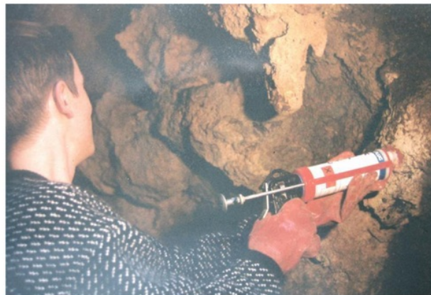
Figure 83. Grout gun in use during restoration at Swiss Garden fernery/grotto.
