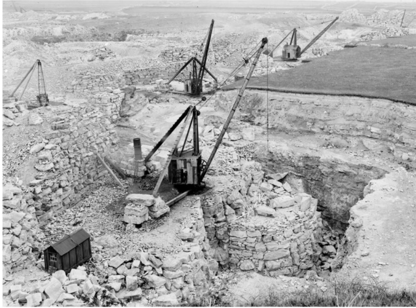
Figure 30. Derrick cranes in use in a Dorset quarry.
