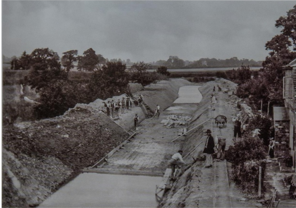
Figure 78. Work on a section of Thames & Severn Canal c1904. Labourers using puddled clay for canal lining.
