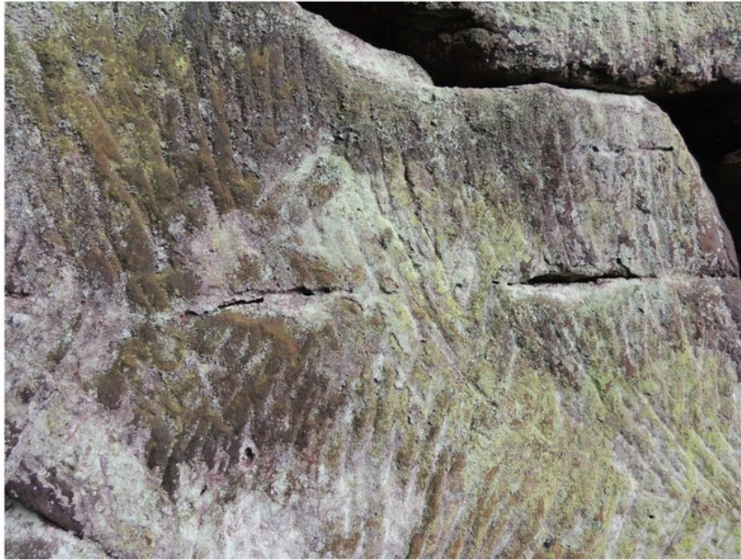
Figure 69. Chisel marks seen on rockwork at Hawkstone Park 2017.
