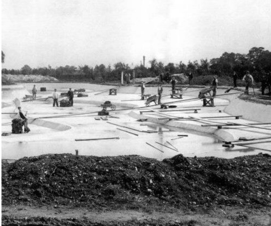
Figure 84. Lake excavation at Burnby Hall gardens 1904. Still using wheelbarrows and planks and basic tools.
