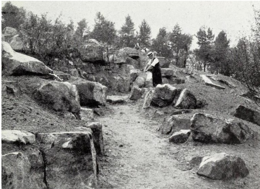
Figure 94. Wisley in the course of construction, 1911.
