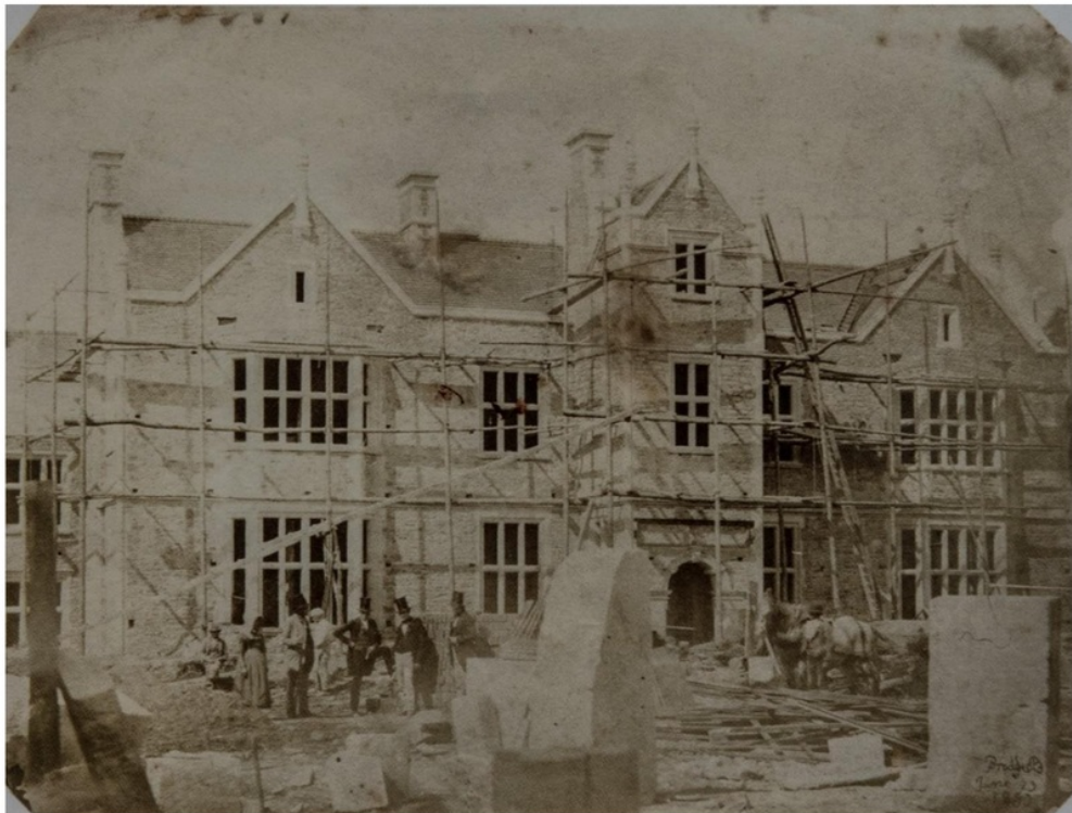
Figure 27. Wooden scaffolding and ladder used in 1853 house construction.
