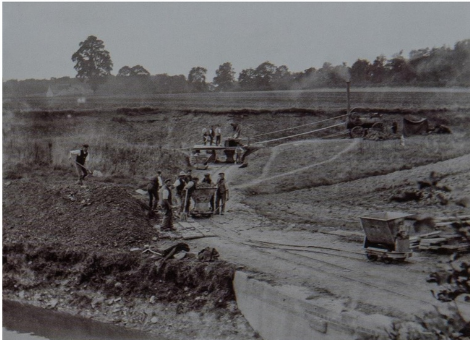
Figure 90. Labourers making puddling clay to provide a watertight lining for Thames and Severn Canal c1904. Note use of temporary railway/tramway, tipping wagons and steam engine.
