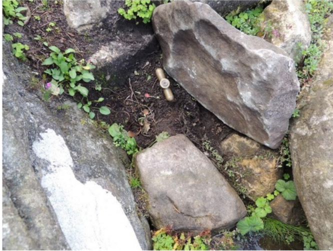
Figure 66. Simple tap at the top of the cascade at Cragside.
