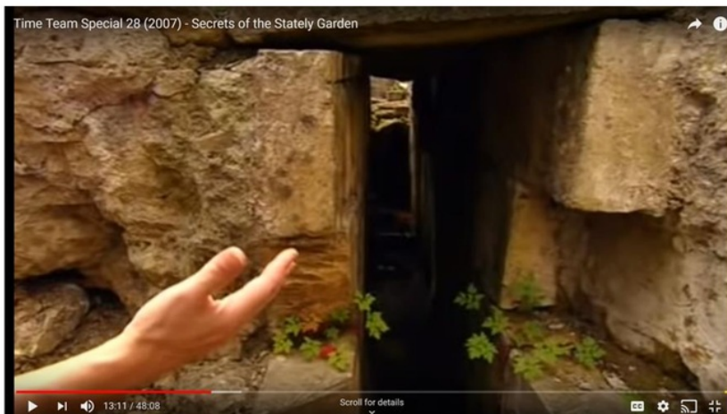
Figure 63. Prior Park – stone culvert found during restoration of the cascade.
