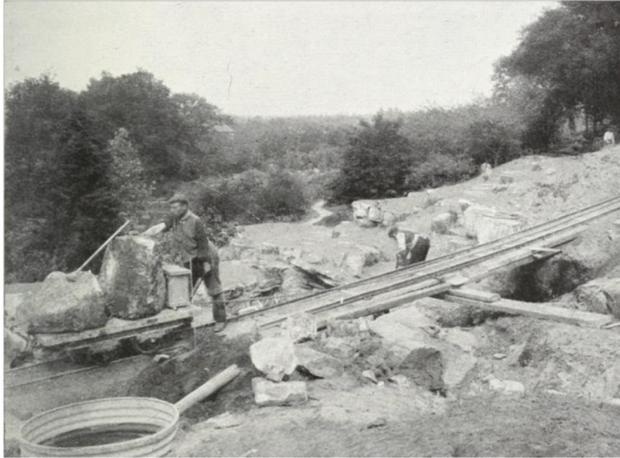
Figure 93. Wisley rock garden during construction. Note use of temporary tramway and low-level wagon to move rocks being guided by hand. Also use of planks for support.
