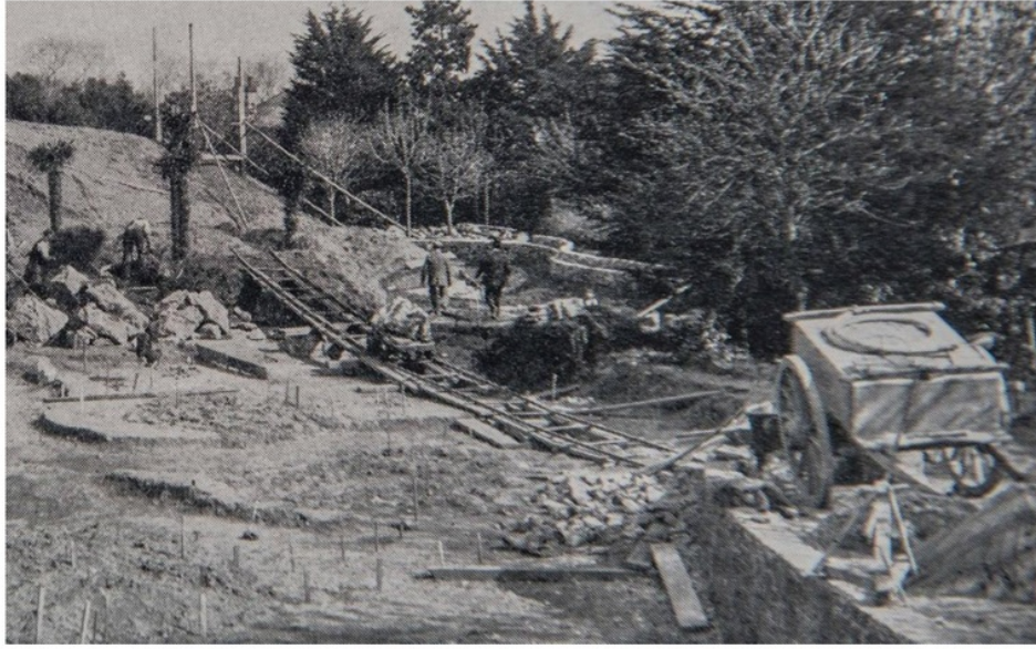
Figure 68. Equipment used by Meyer on a site in Paignton. Note the pegs for laying out (foreground), temporary rails and trolley, wheelbarrows.
