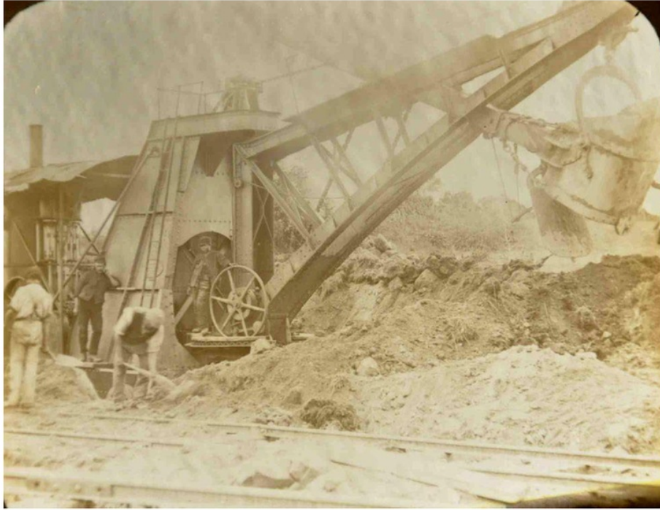
Figure 34. Steam-driven trencher in 1880s, used in Katrine aqueduct construction, Scotland.
