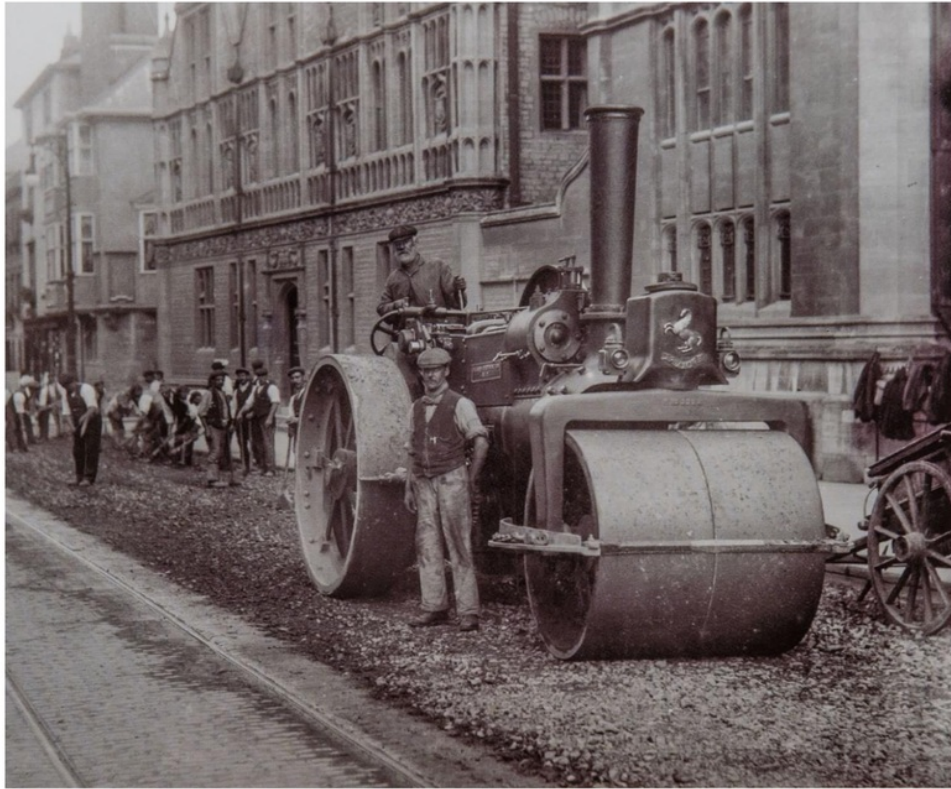
Figure 35. Labourers laying substrate of new macadam road surface with the aid of a steam roller, Oxford c1900.
