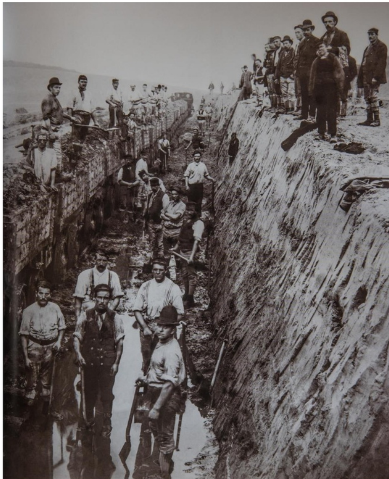
Figure 92. Hand excavation of Manchester ship canal c1889. Note use of temporary railway for removing spoil.
