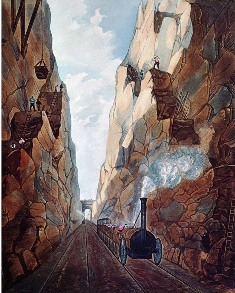
Figure 39. T. T. Bury, Excavation of Olive Mount, 4 miles from Liverpool, 1831 . Note the navvies hacking the rock with pickaxes.
