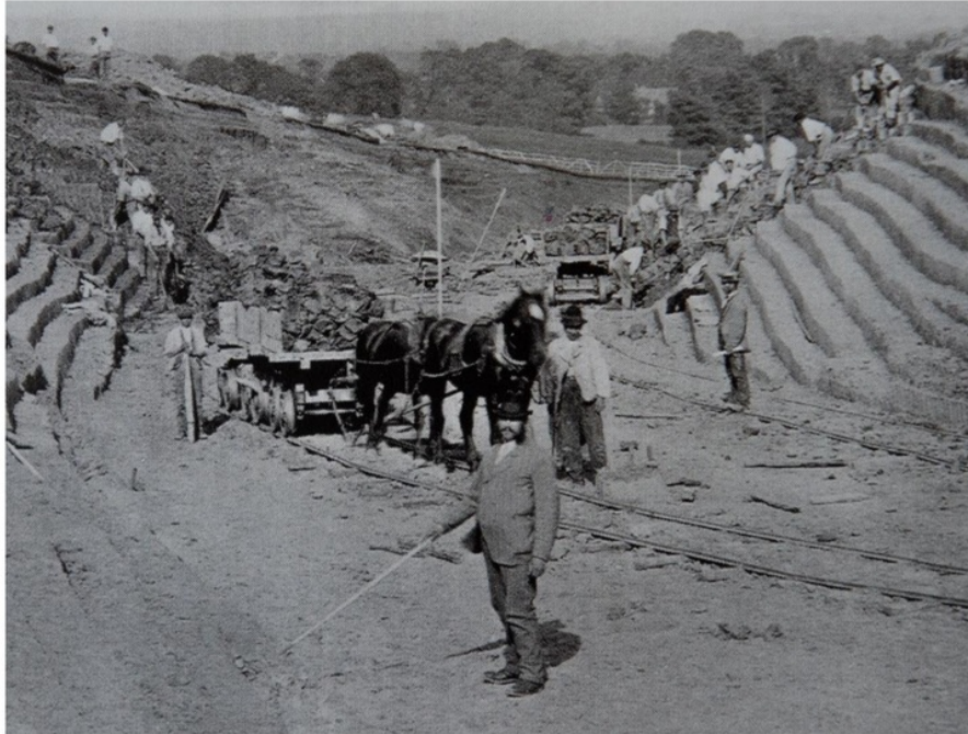
Figure 53. Excavation work at Waddesdon. Note the horse and cart, tramway and use of pick-axes and shovels.
