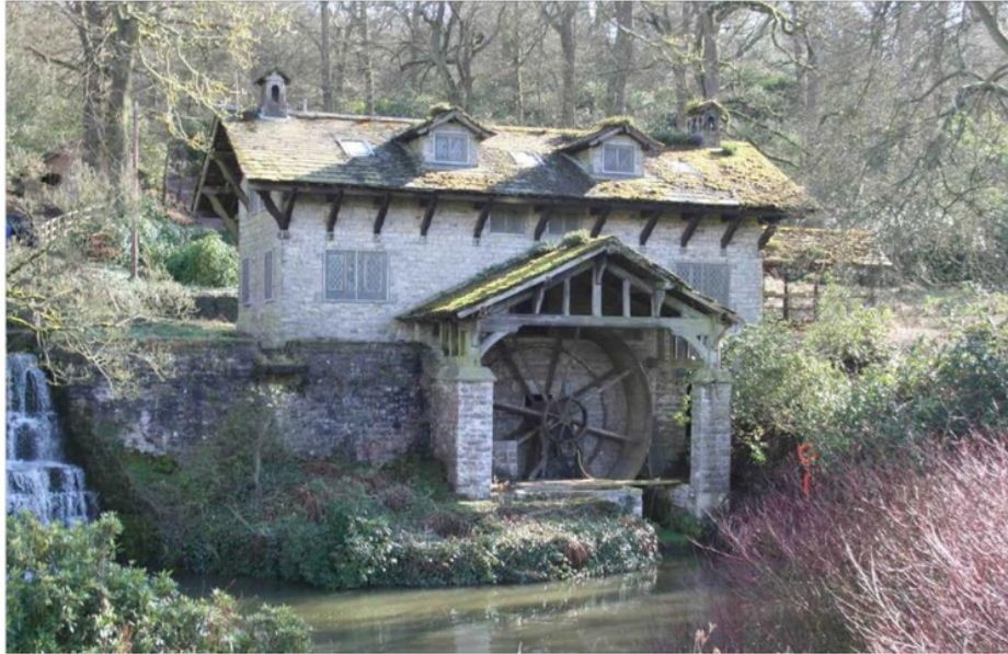
Figure 61. Pump house at Osmaston Manor. The cascade is on the left.
