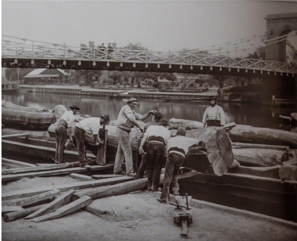
Figure 19. Workmen load large logs onto a river barge using a jack (centre of picture, jack operated by 2 nd man from left). A second jack lies on the canal edge.
