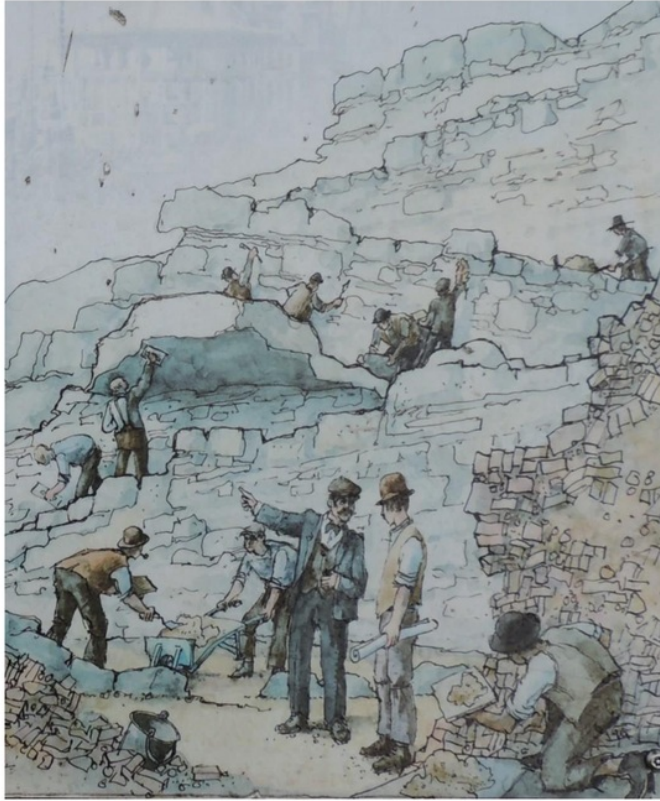
Figure 79. Artist's image of Pulham's men constructing the Zig-zag path at Folkstone. Note the wheelbarrow, bucket, hawk and finishing trowel.
