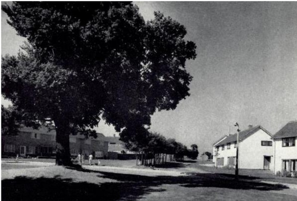
Figure 44: Existing trees are incorporated into new housing development in Basildon. Source: Sylvia Crowe, Tomorrow's Landscape (London, The Architectural Press, 1956), p. 25.
