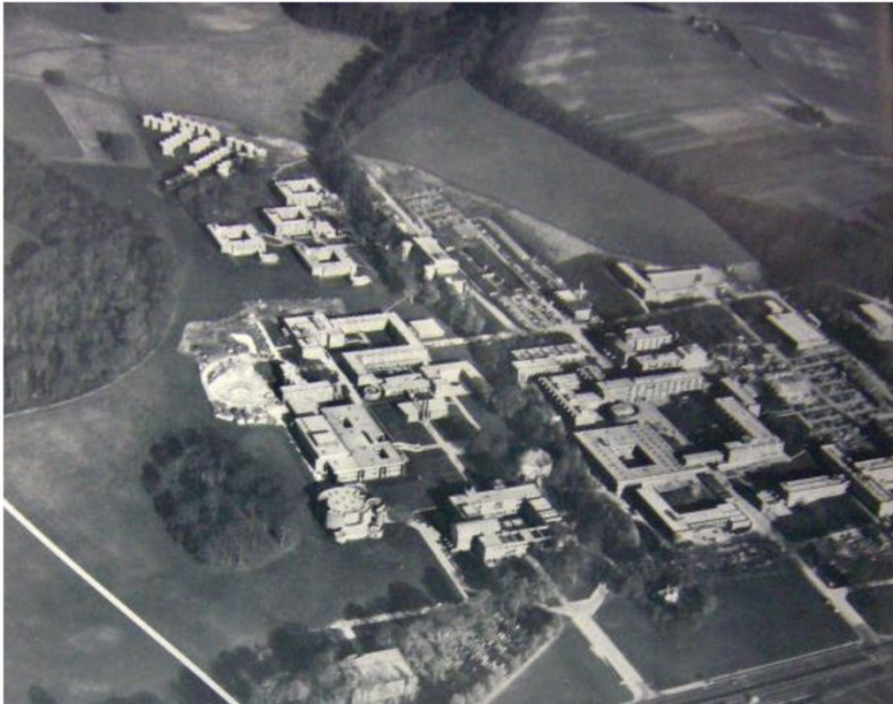
Figure 45: Aerial view of the University of Sussex from the southwest c. 1973. Source: HES AR BS, SX UOS 1/1/15/3.
