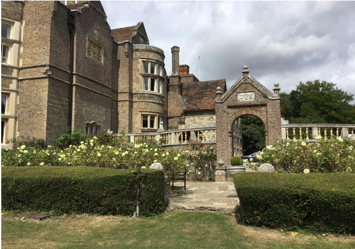
Fig. 95. The courtyard at Betteshanger House 2019.
