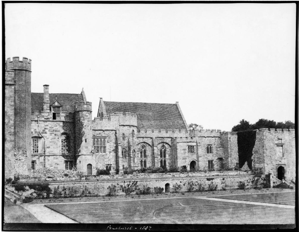
Fig. 78. Penshurst Place 1857, note the pile of rubble where the curtain wall had been removed and the plain lawns. Historic England DD67/00047 .
