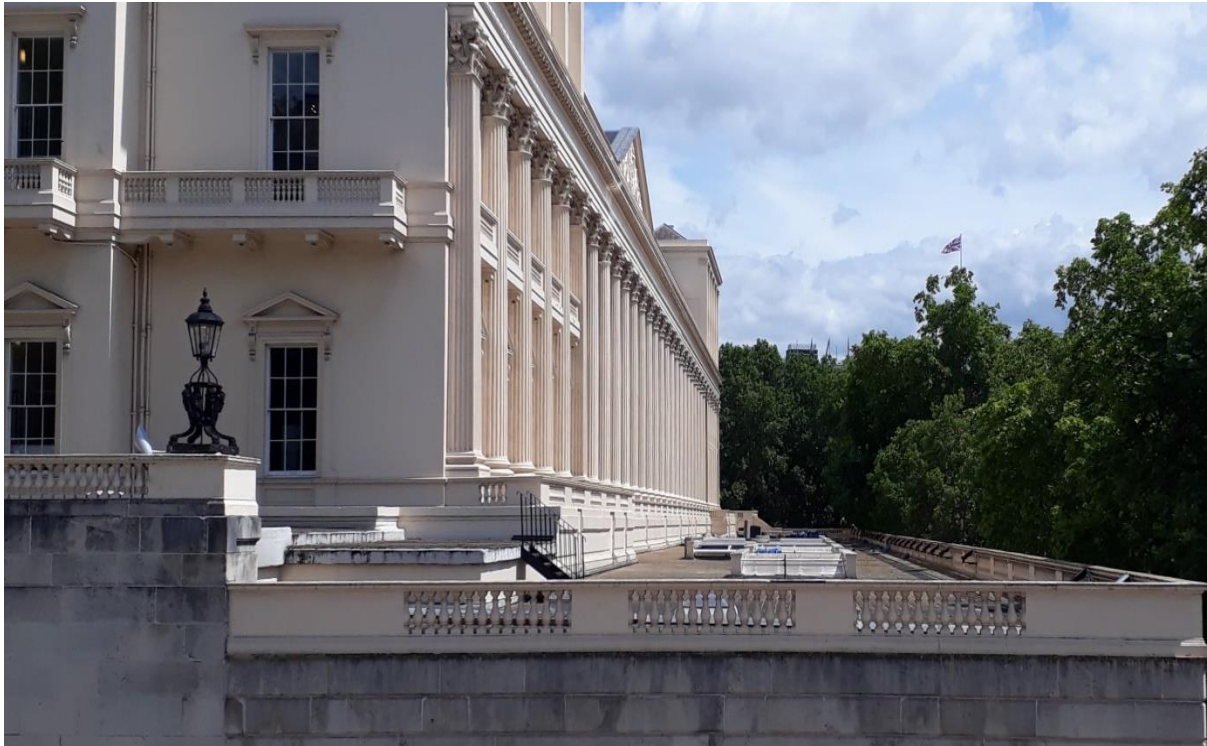
Fig. 201. Carlton House Terrace, the eastern side looking towards the site of Lord Granville's garden at the end of the Podium, 2019.
