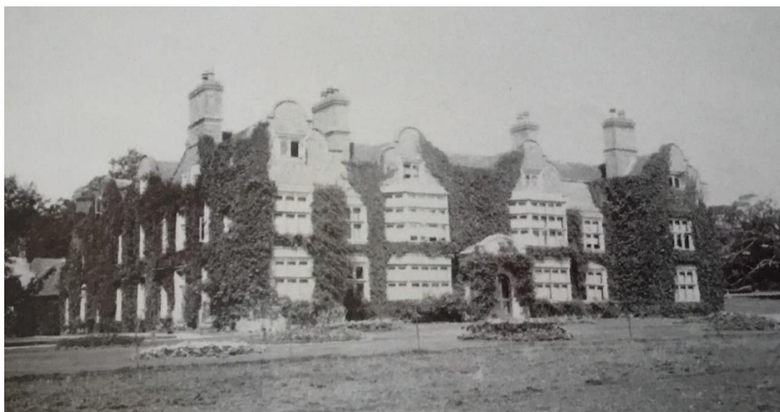
Fig. 224. Godinton circa 1870s, a layout of circular flower beds. The Godinton House Preservation Trust .
