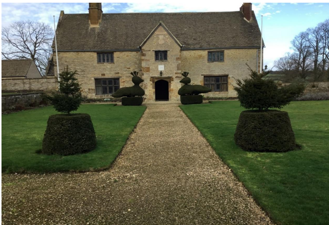
Fig. 378. Through the gate to the front of the Manor. 2020.
