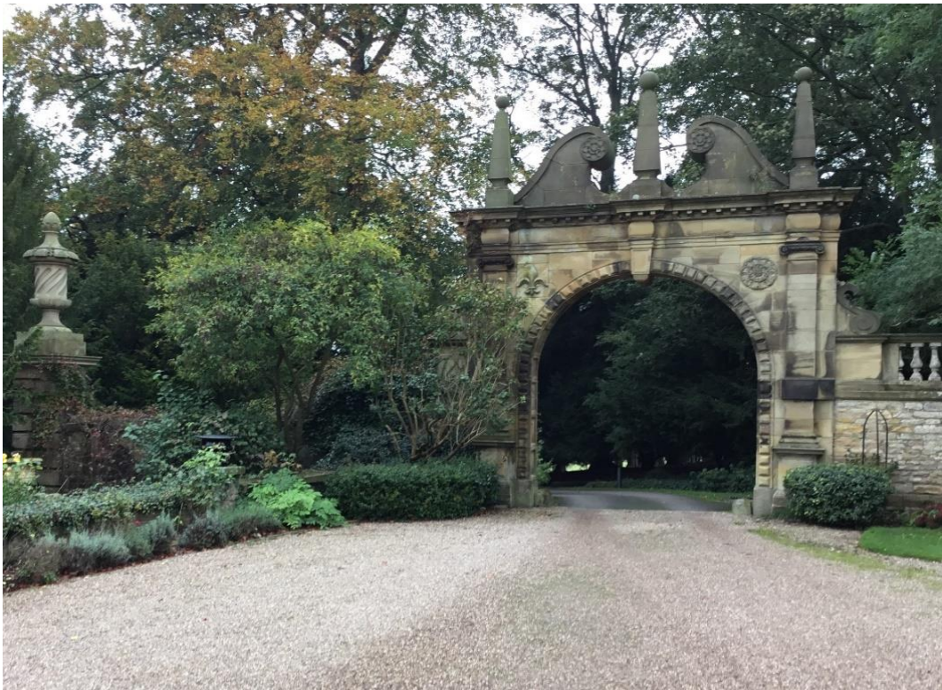
Fig. 172. Brantinghamthorpe Hall, the archway. 2019.
