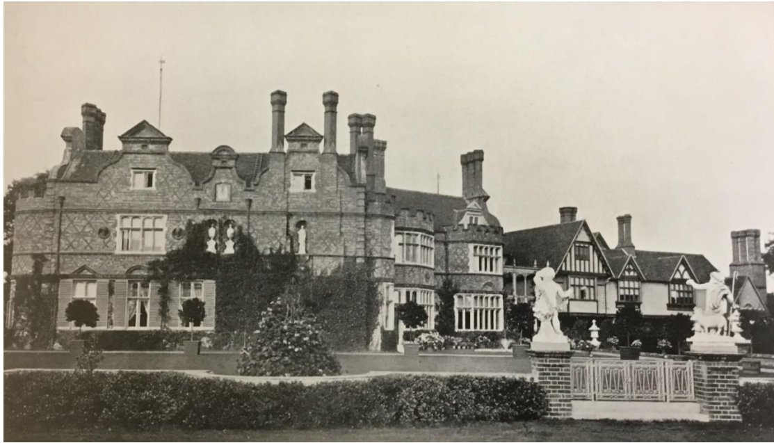
Fig. 103. Coombe Warren House, note the diapered brickwork, alcoves and tondos. The Work of George Devey Architect , no date.
