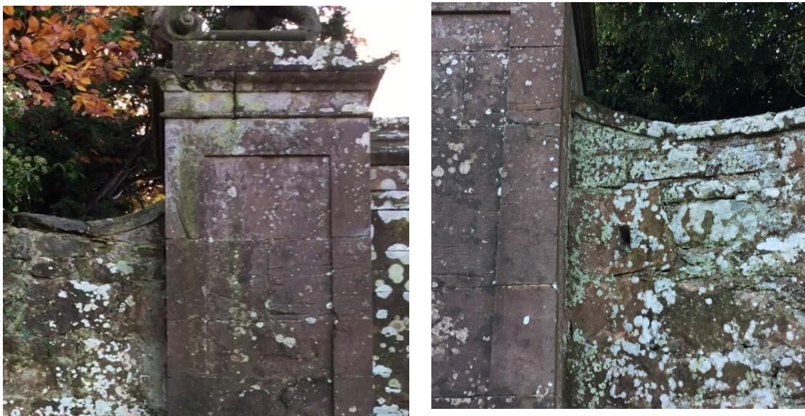
Fig. 144. The entrance wall, piers and gateway at Condover Hall showing the growth of lichen. 2019.
