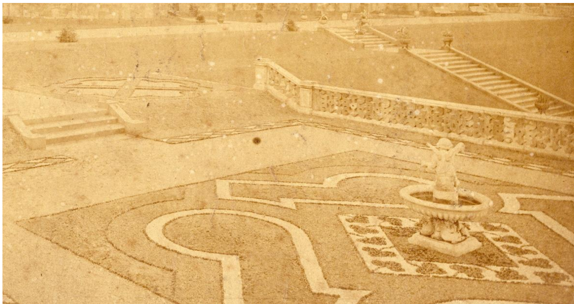
Fig. 118. A similar parterre design by Devey at Killarney House, circa 1870s. RIBA 114989.
