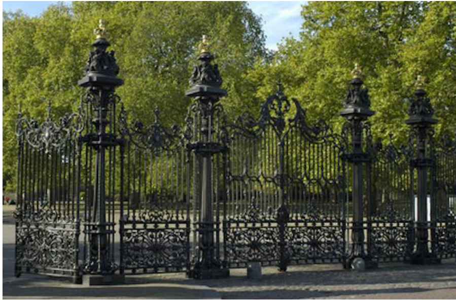
Figure 38. Coalbrookdale cast iron gates at Kensington Gardens. Jennie Hills, 2003, Science and Society Picture Library.
