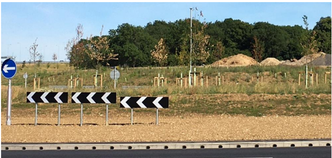
Figure 30. Sheering Road roundabout, Harlow, 07/2022.
