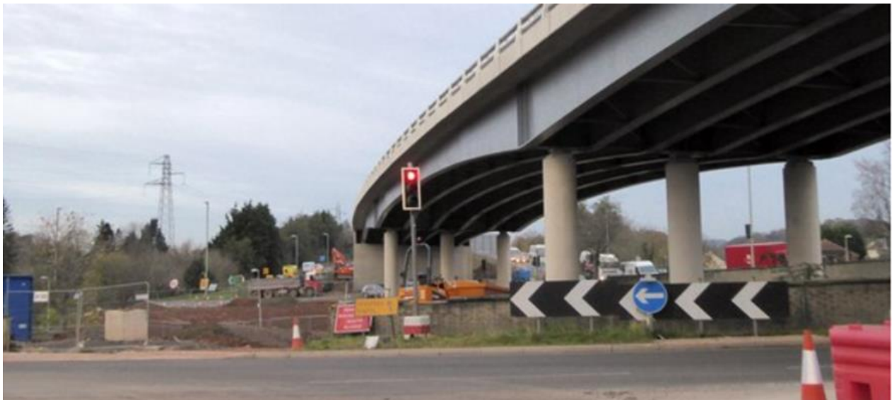
Figure 52. Penn Inn roundabout, Newton Abbot, prior to community work, 2017.
