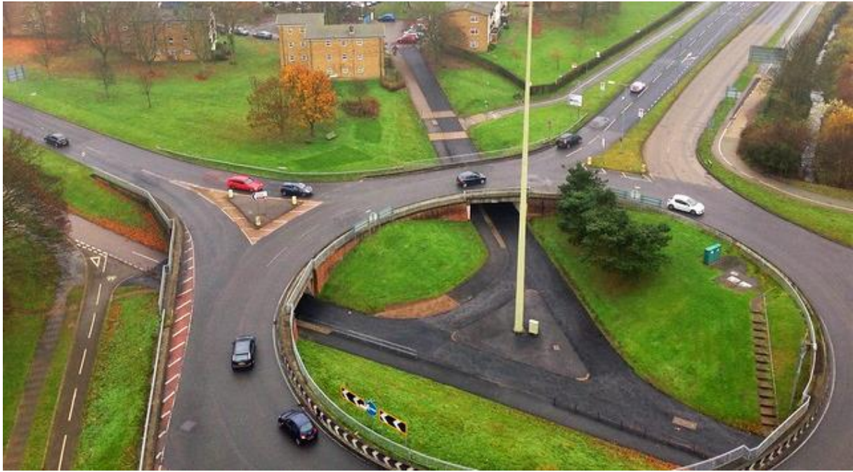
Figure 32. Six Hills Way ‘doughnut’ roundabout, Stevenage, nd.
