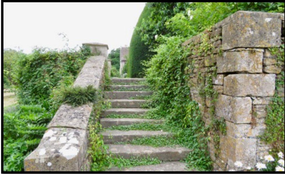
Figure 3.72: Steps and Dry Stone Wall (2017)
