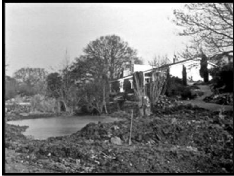
Figure 62: White Barn, A Pond under Construction (1960s)
