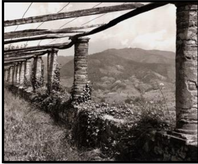
Figure 13.60: Cleared Vine Pergola (1960s)
