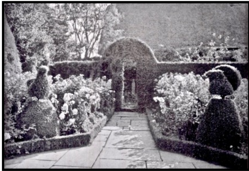
Figure 4.31: Old Garden Paved (1930)
